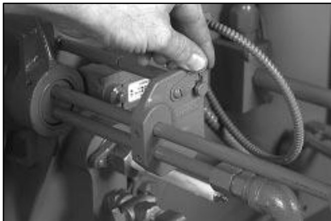
Figure: 5-13 Oil Gun Locked in OUT Position
