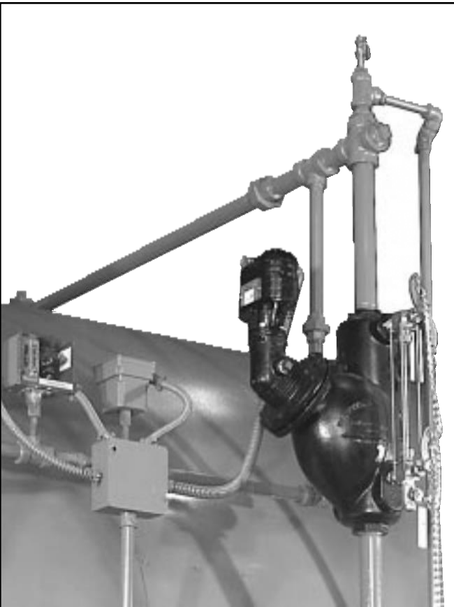
Figure: 1-4 Low Water Cut Off (LWCO)
