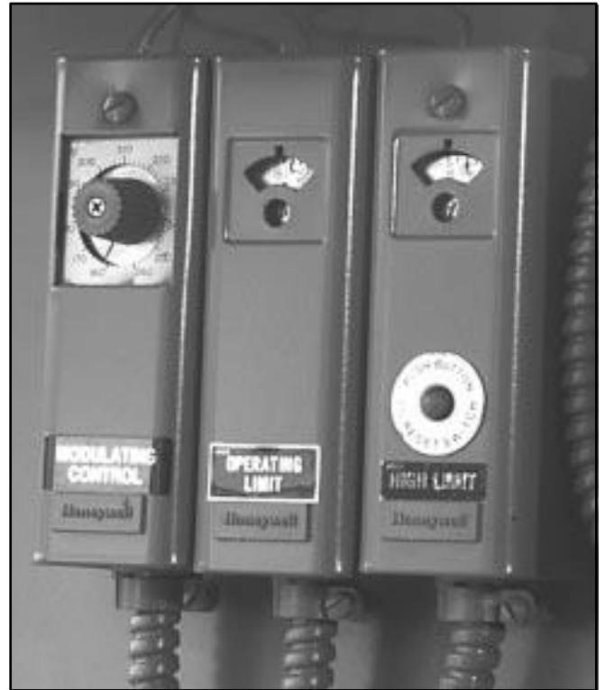
Figure: 1-12 Hot Water Controls
