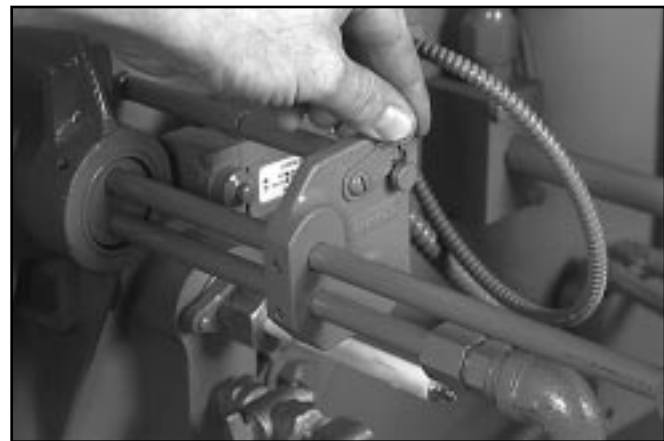
Figure 6-18 Oil Gun Locked Out
