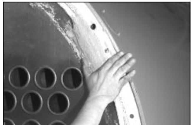
Figure 8-30: Apply Pulp Over Rope and Tadpole Gasket
