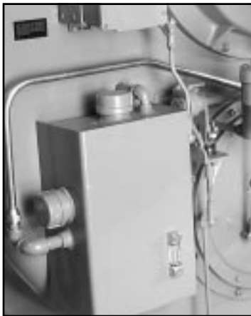
Figure 8-20: Air Oil Receiver Tank CB-LE
