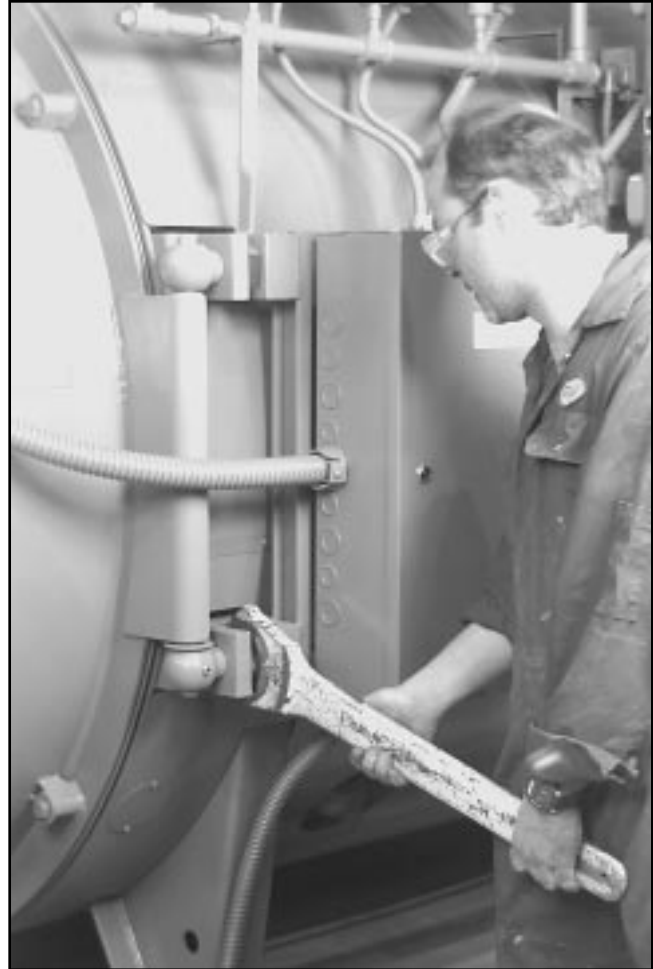
Figure 8-36: Tighten Hinge Bolts
