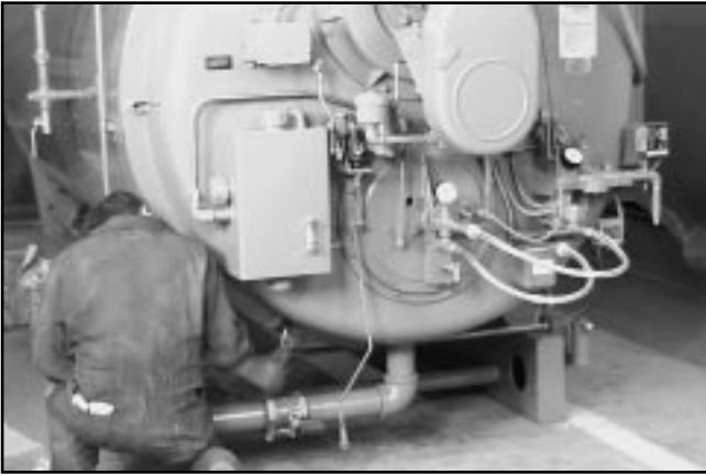
Figure 8-35: Close and Tighten Front Head
