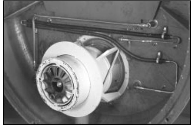
Figure 8-33: Inspect and Clean Inside Front Head and Components
