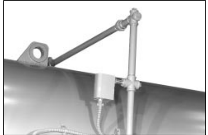
Figure: 1-13 Low Water Cutoff (LWCO Hot Water)
