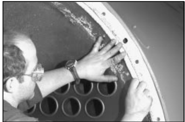
Figure 8-29: Rope Gasket Glued against Tadpole Gasket
