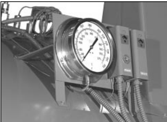
Figure: 1-11 Water Temperature Gauge
